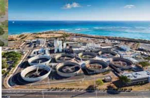
Sand Island Wastewater Treatment Plant Secondary Treatment Ph 2
