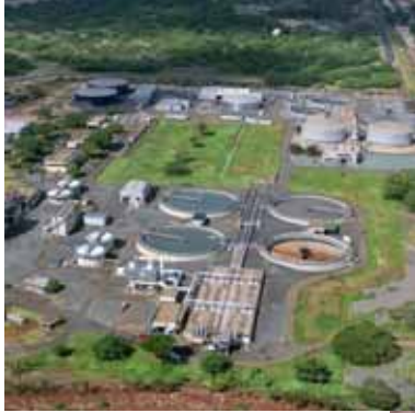
Honouliuli Wastewater Treatment Plant
